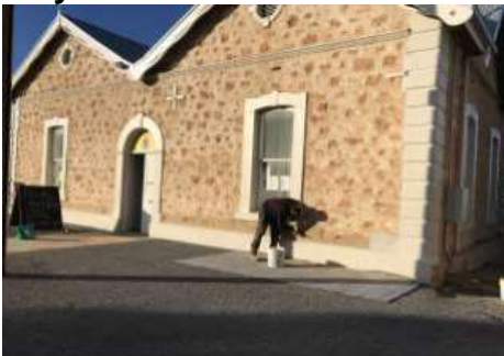
Newsletter Building/ Former Port Wakefield Council Office stone repointing carried out
